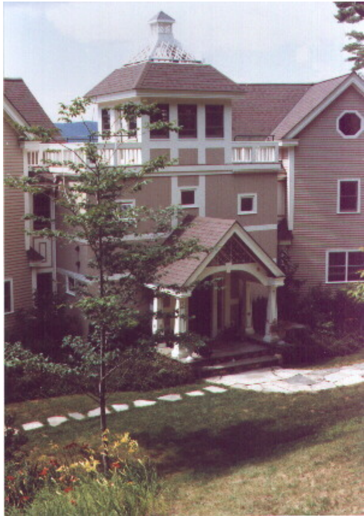
Entry Façade View
