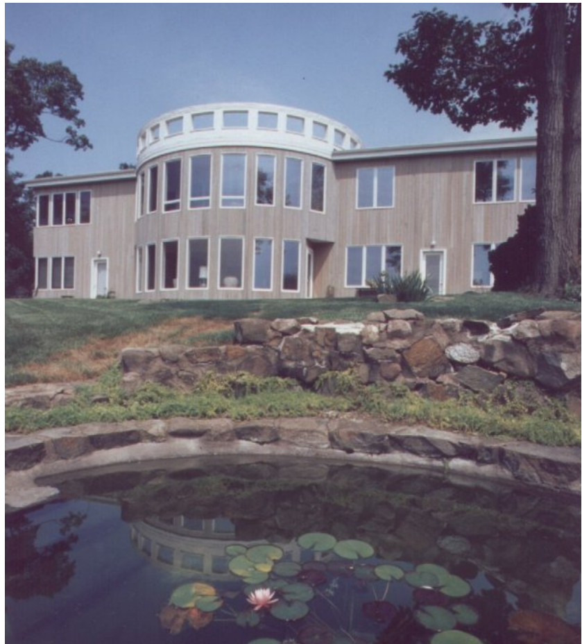
Exterior After Renovation
