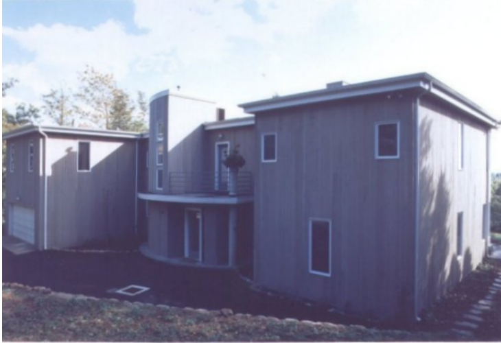
Exterior Before Renovation
